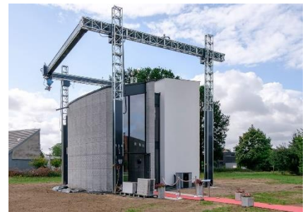
Figure 11. House construction printing with a 3D printer
