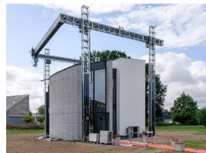
Figure 11: House construction printing with a 3D printer
